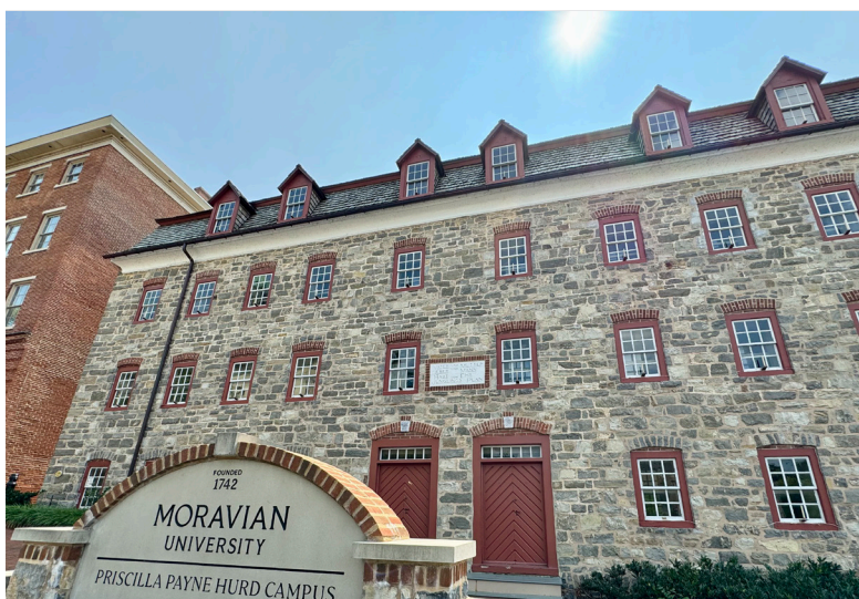
Second Single Brethren's House in Bethlehem
